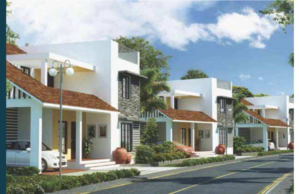
ERBIL LIME LIGHT HOUSING PROJECT 1000 VILLAS ERBIL IRAQ 2010-2011
