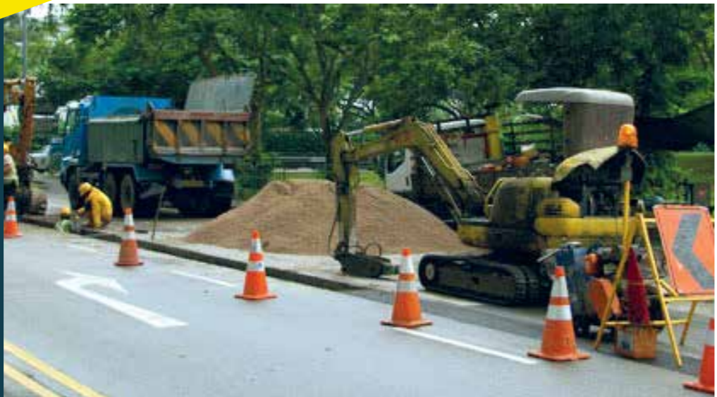
ASPHALT CONSTRUCTION WORK TRIPOLI
