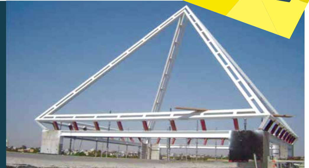
CONCO HEADQUARTER BUILDING AT AHMADI 2006
