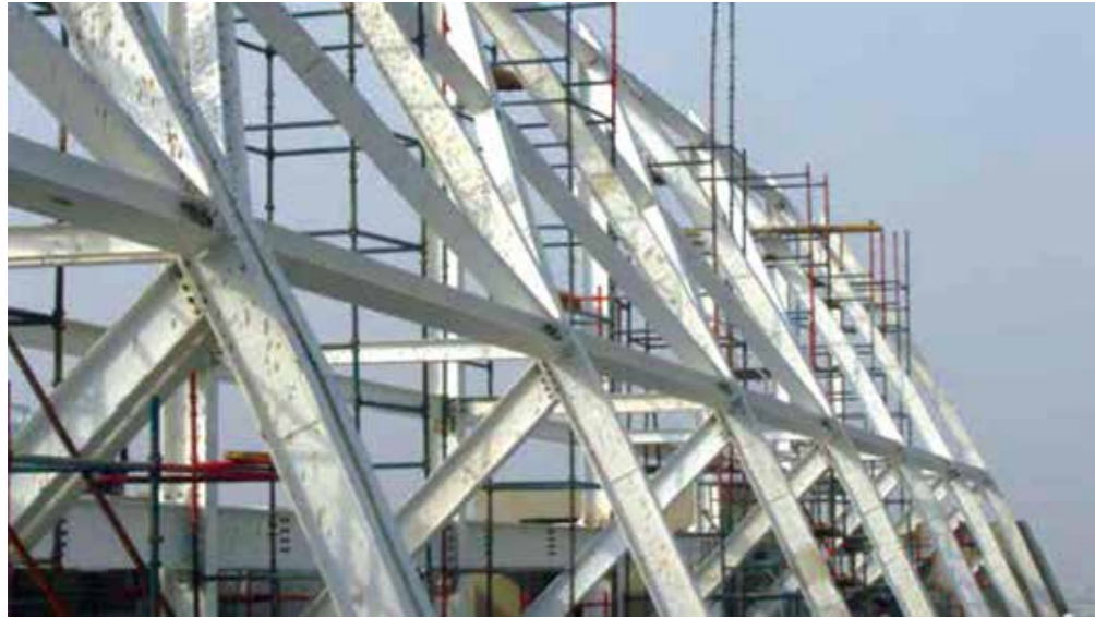
KUWAIT OIL TANKER COMPANY MAIN OFFICE BUILDING 2009
