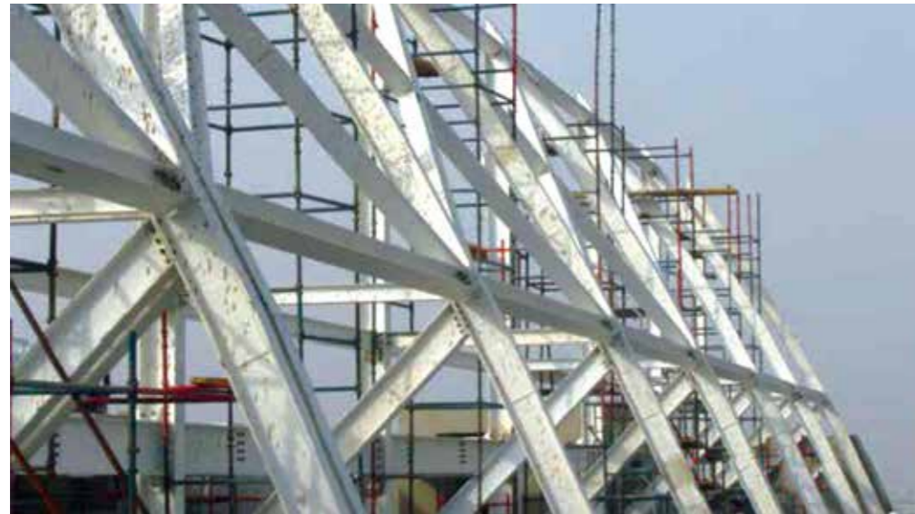
KUWAIT OIL TANKER COMPANY MAIN OFFICE BUILDING 2009
