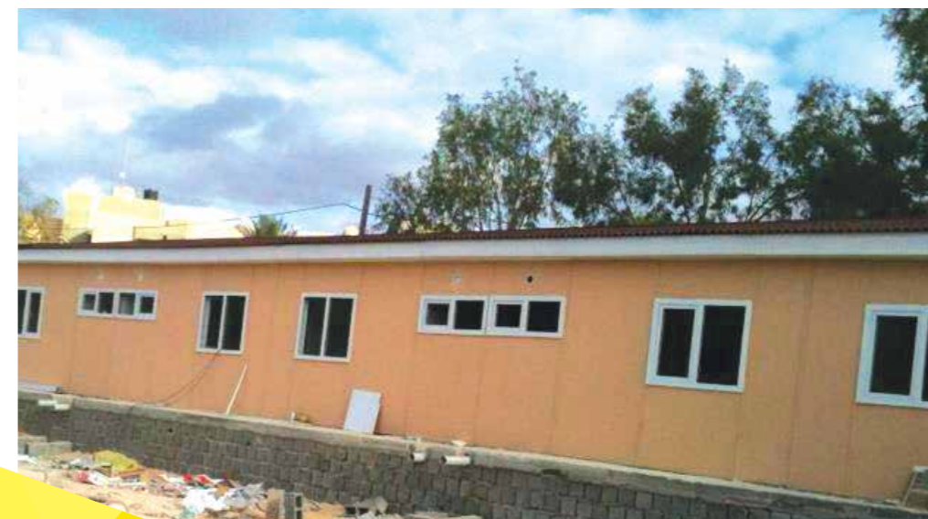
MUSIRATA HOSPITAL SITE OFFICES PROJECT
