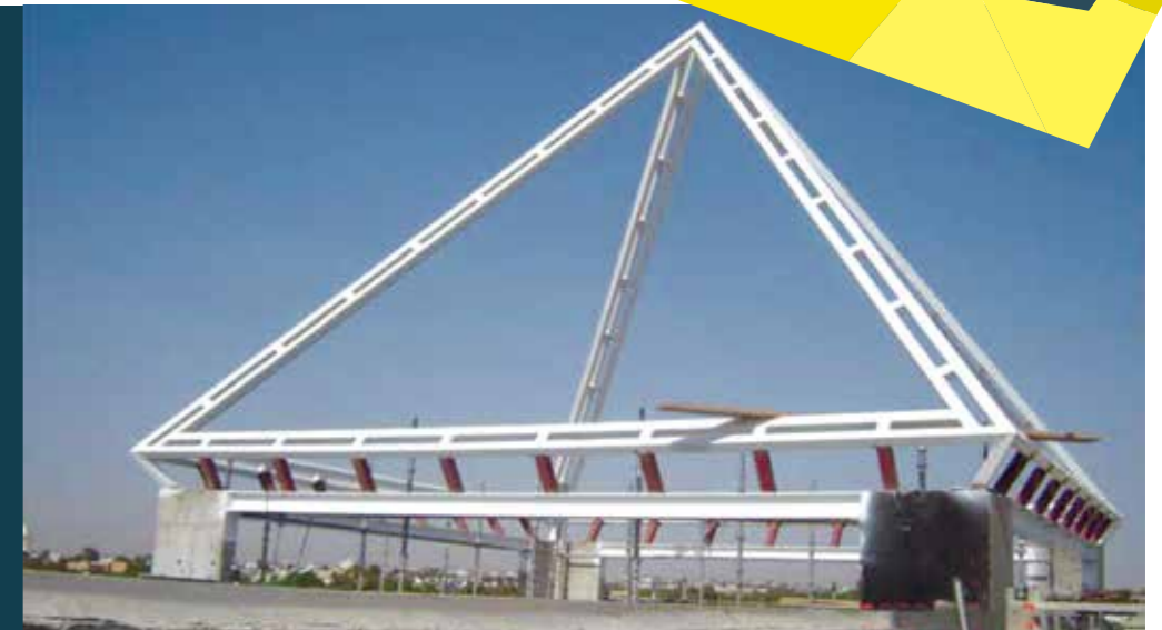
CONCO HEADQUARTER BUILDING AT AHMADI 2006
