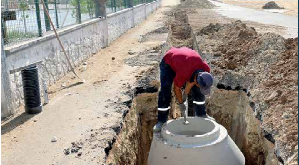
ASPHALT CONSTRUCTION WORK
