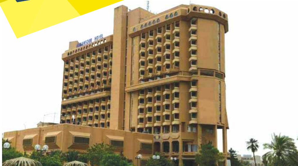
MANSOUR MILYA HOTEL RENOVATION PROJECT BAGHDAD 2010-2011
